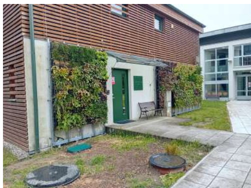
Fig. 3: Teaching interactive model – green facade and rainwater retention tank (Source: photo by author)
