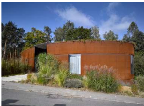
Fig. 10.: Family House "Heart" – street façade with curvature and landscape integration (Source: https://www.archiweb.cz/b/rodinny-dum-srdce )
