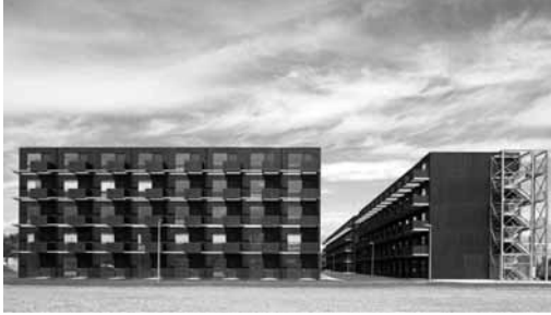
Fig. 3: The dark façade of the hall of residence in Zuiderzeeweg is strictly composed of repeated dwelling modules (Source: FRIEDMAN, A. Innovative student residences: new directions in sustainable design, s. 49.)
