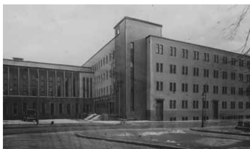
Fig. 5. "Dom Żołnierza" in Poznań, 1939, design and rebuilt after war by Władysław Czarnecki (1939) (source: NAC, sign. 1-W-1052-1)
