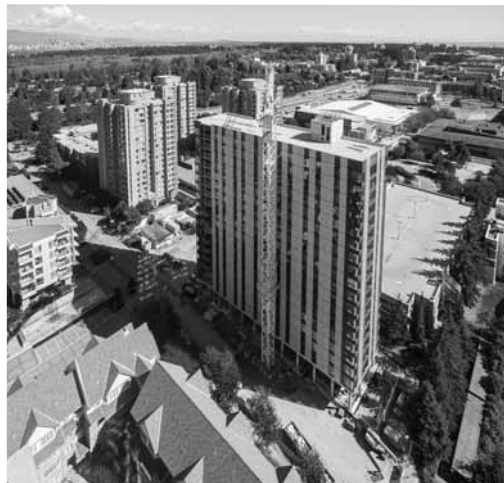
Picture 1.: Eighteen floor building with the structure based on wood using CLT panels, Vancouver (Source: www.archdaily.com)
