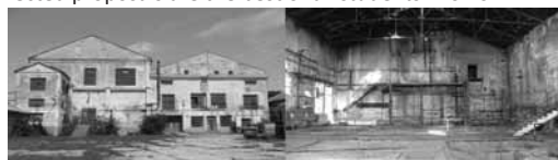
Fig. 6: Original condition of ammunition factory (Source: Monumental board in Komárno)
