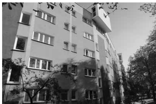
Fig. 2.: Juliusz Słowacki housing estate in Lublin designed by Oskar and Zofia Hansens (1960–1963) (Source: photo by Mariusz Zadworny)
