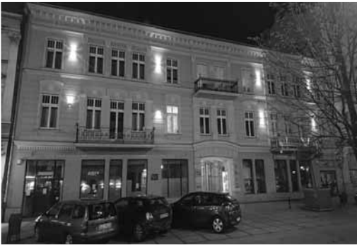
Fig. 2.: Tenement house in Częstochowa Al. NMP 33 with modest illumination, however location of sources of light is „accidental” and not reflecting architectural division of the façade. Author: S. Wróblewski 2018.
