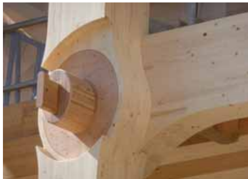
Obr. 4: Detail spoje ( https://www.archdaily.com/478633/tamedia-office-building-shigeru-ban-architects/5304250be8e44ef683000d2-tamedia-office-building-shigeru-ban-architects-image )
