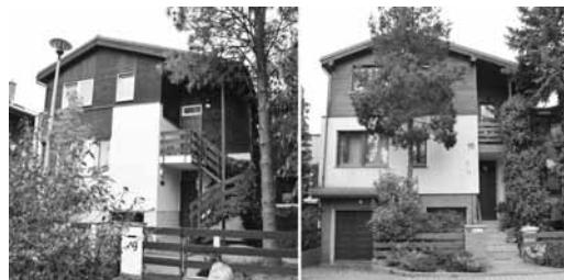
Fig. 4: Example of a building with a superstructure, completed according to the Proj. of L. Konarzewski (source: photo Z. Napieralska)
