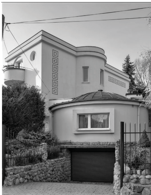
Fig. 8 Example of uncontrolled modernization of a dome building at ul. Ustrzycka in Warsaw (source: www.fotopolska.eu)
