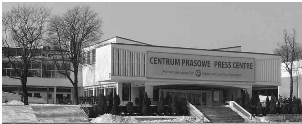
Fig. 4. the Ministry of Transportation Hall, Poznań International Fair, design by Bolesław Szmidt (1949) (source: https://pl.wikipedia.org/wiki/Pawilon_Ministerstwa_Komunikacji_na_MTP , accessed: 18.09.2018)
