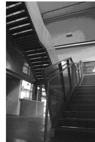
Pic.: 16: steel staircase
