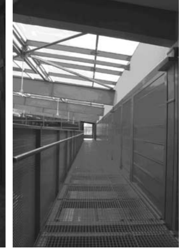
Pic.: 15: accessory balcony along the lobby
