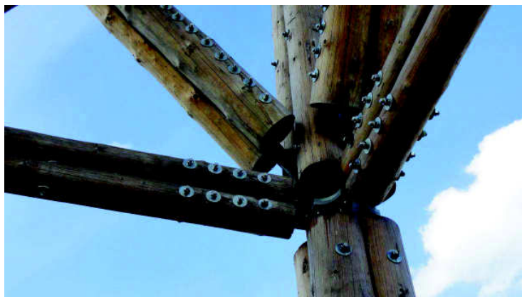
Fig. 8 Example of a round timber bolted joint with slotted-in steel plates
