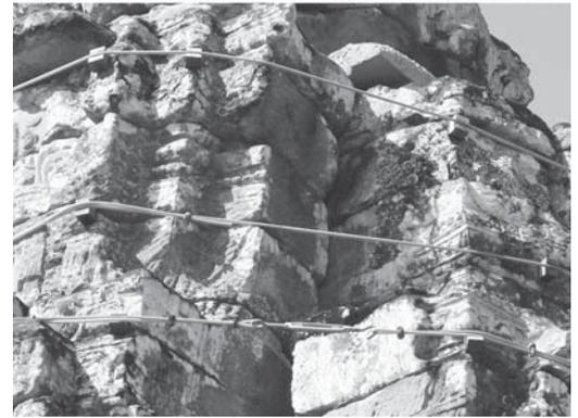
Fig. 12.: Sealing of vault joints of Angkor Wat temple gallery in order to prevent leakages of rainwater by application of lead foils and sheets; stabilisation of tower of Preah Khan temple by means of prestressed rings (Source: author)
