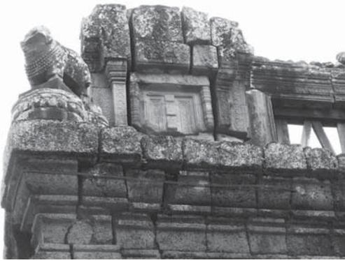
Fig. 8.: Typical failures of stone monuments – progressive collapse of gallery structure of Ta Prohm temple; open joints between the laterite blocks at corner loaded by the statue (Phimeanakas temple) (Source: author)
