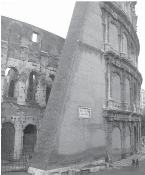
Fig. 5.: The Colosseum in Rome. Retaining wall and arcades rebuilt from years 1805 - 1807. Architects Palazzi, Camporese and Stern (Source: author).
