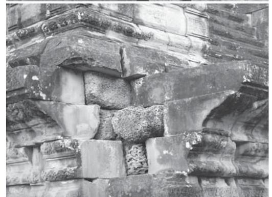
Fig. 7.: Signs of stonework disintegration – delamination of sandstone columns of the Angkor Wat gallery; defragmentation of stonework made of sandstone and laterite blocks (pyramid of Angkor Wat temple) (Source: author)
