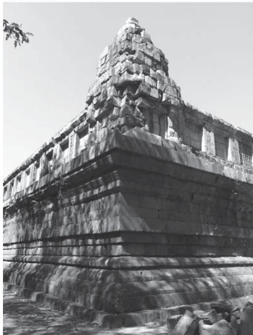
Fig. 11.: The pyramid corner of Ta Keo temple damaged by expansion movements of the stonework and as a result of overloading by the tower – the condition before and after the reconstruction according to the method of addition of newly fabricated laterite stone blocks (Source: author)
