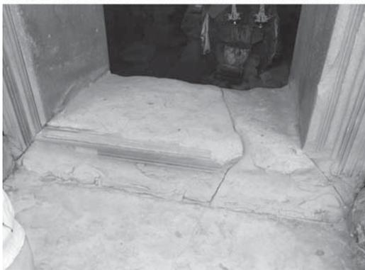
Fig. 9.: Crack in the brickwork of a tower (Bakong temple); broken sandstone doorsill of brick wall, being pushed into the subgrade on the sides (Pre Rup temple) (Source: author)
