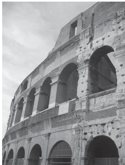
Fig. 7.: The Colosseum in Rome. Rebuilt arcades of color-coded bricks, executed arch. L. Canina in the years 1840-1852. (Source: author)
