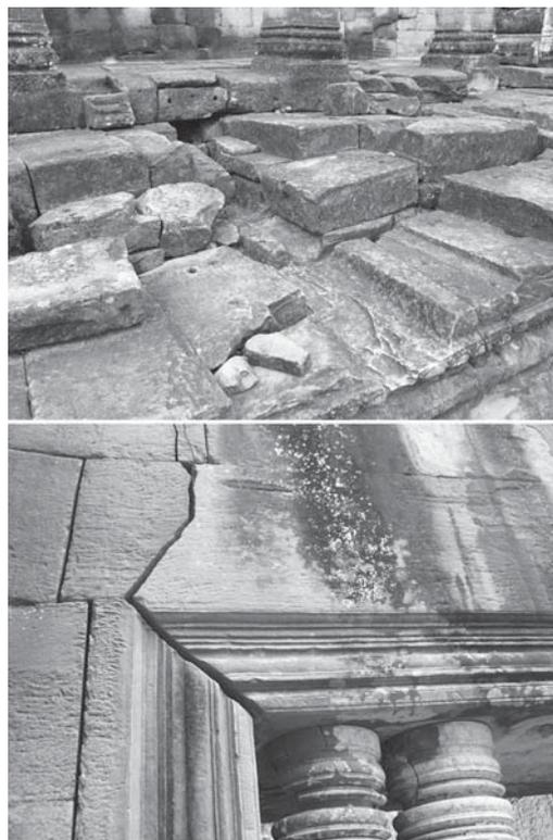
Fig. 4.: Damaged system for rainwater draining from the pyramid terrace of Bayon temple; conical shape of mating surfaces of sandstone blocks edging the openings of Ta Keo temple (Source: author)
