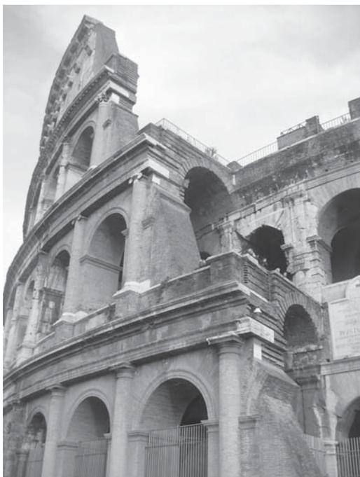
Fig. 6.: Colosseum in Rome. Retaining wall in the shape of the original arcade, G. Valadier realized in the years 1823 - 1826 (Source: author)
