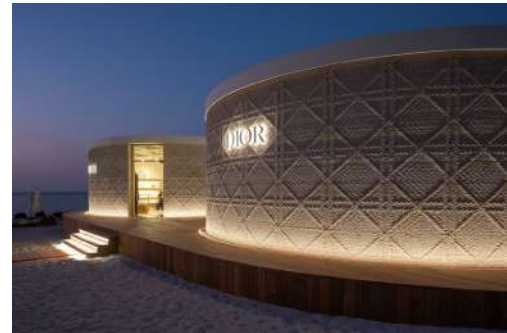
Fig. 10.: 3D Printed Earthen Pavilion for the fashion company Dior. (Source: 3D WASP, 2021 Concept store Dior, 2021. In: 3D Wasp [online]. Italy: 3D Wasp Available from: https://www.3dwasp.com/en/3d-printed-pop-up-store-wasp-dior/ [Accessed June 30, 2023])
