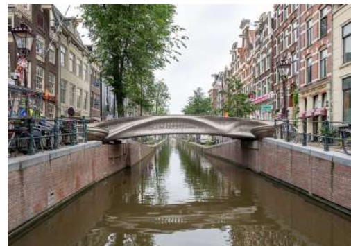
Fig. 6.: Metal bridge created using 3D printing. (Source: MX3D, 2019 Smart bridge (Source: Smart bridge, 2019. In: MX3D [online]. Amsterdam: MX3D. Available from: https://mx3d.com/industries/design/smart-bridge/ ) [Accessed June 30, 2023])
