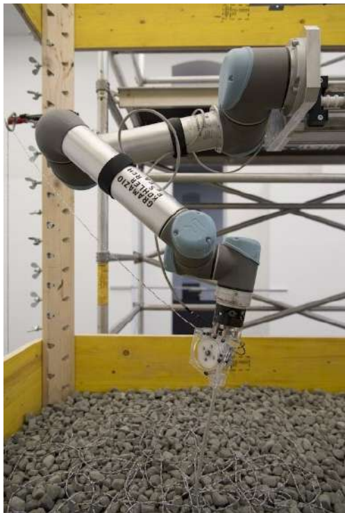
Fig. 5.: Additive manufacturing using reversible concrete. (Source: MIT, 2015. Reversible Concrete. Web urbanist. Available at: https://weburbanist.com/2015/10/10/reversible-concrete-3d-printing-for-easy-deconstruction-reuse/ [Accessed June 30, 2023])
