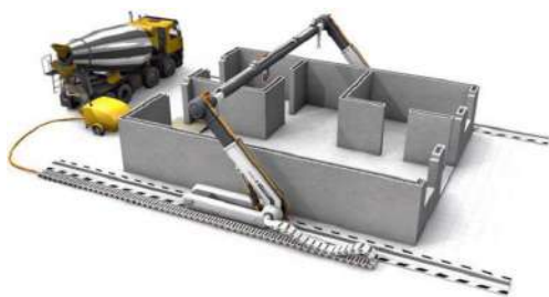
Fig. 1.: Printing technology Countour. (Source: Crafting, C., 2017. Countour crafting for space application. Countour crafting. Available at: https://www.countourcrafting.com/space [Accessed June 30, 2023])
