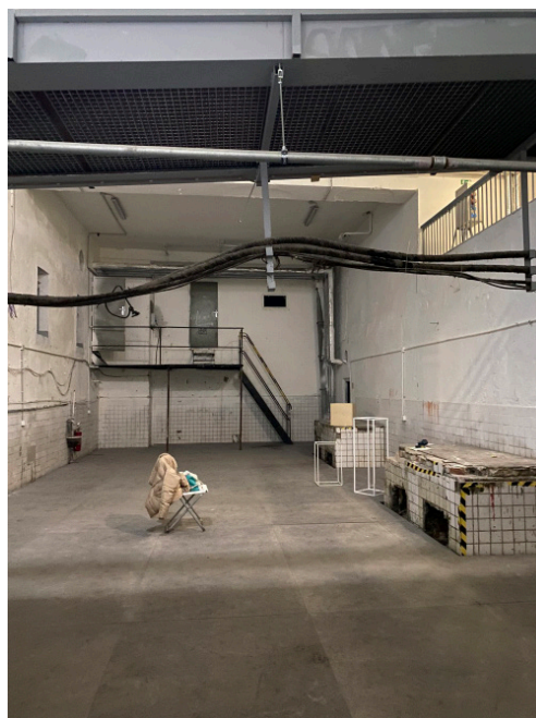
Fig. 1.: Boiler room space at FAD STU BA. (Source: author)
