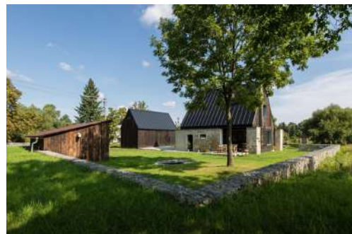
Fig. 12.: The construction of the house is inserted into the furthest part of the original building. (Source: TŘI.ČTRNÁCT architects)
