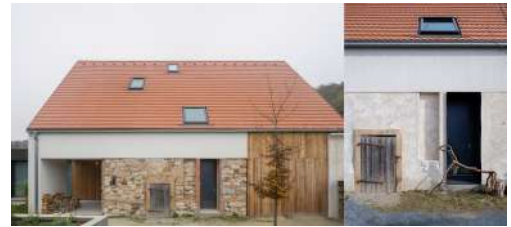
Fig. 5.: Photo from the official presentation (left) compared to the state in 2022. A fragment of the stone wall was plastered using traditional technology. This solution is less spectacular than the presentation of exposed masonry and preserves the authenticity of the original building. (Source: projectstudio8, Pavel Fuchs)
