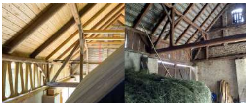
Fig. 7.: Comparison of the barn in Loubí before and after renovation (left). The planking has been replaced with carved wood. The purpose was to lighten the space, but the solution remotely resembles the ornaments of folk architecture. (Source: atelier SAD)
