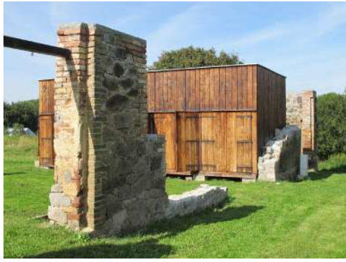
Fig. 2.: The ruins of the barn around the object in Verneřice were partially refilled and stabilised by the authors. (Source: Labor13)
