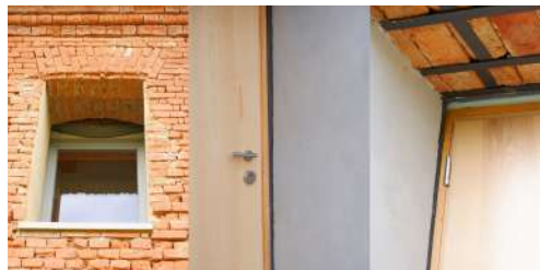
Fig. 9.: Detail of window and door openings in Arnořtov. Air gap between old and new wall is covered with a protection net. (Source: Pavel Fuchs)
