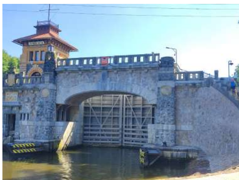
Fig. 3.: The lock of the lock chambre with the Hořín bridge and hydroelectric power plant, part of the Vraňansko – Hořín navigation canal cultural monument. The profile of the lock chamber no longer fits the dimensions of contemporary ship assemblies. The preservation of the structure was achieved by technically demanding widening of the bridge span by 1 m and increasing the underpass height by building a unique hydraulic system to raise one of the spans of the historic bridge by 5 m. (Source: authors)
