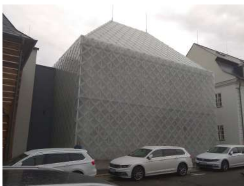
Fig. 8.: Administrative and development building of LASVIT Nový Bor. Two existing heritage-protected houses were renovated using traditional methods, and supplemented by two new ones, materially respectful of the surroundings, but completely modern and futuristic in terms of material and shape. Their surfaces are translucent glass templates in one case, and black cement templates in the other. (Source: authors)
