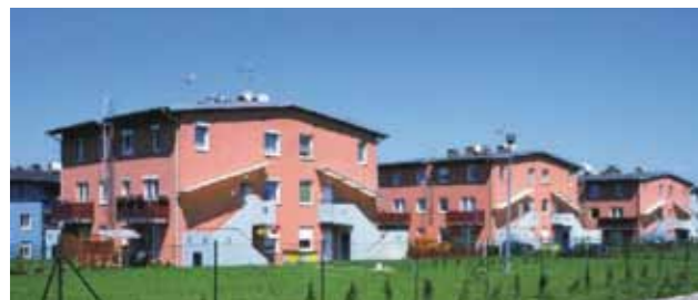
Fig. 3a. The housing complex in Mikołów at Stolarska Street, constructed 2000 – 2002.
