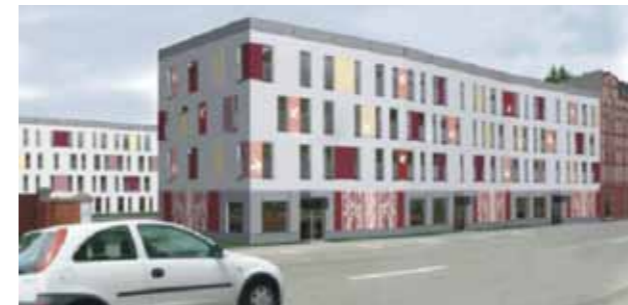
Fig. 6. The housing complex in Katowice at Dębowa and Sportowa Streets. Under construction from 2008
