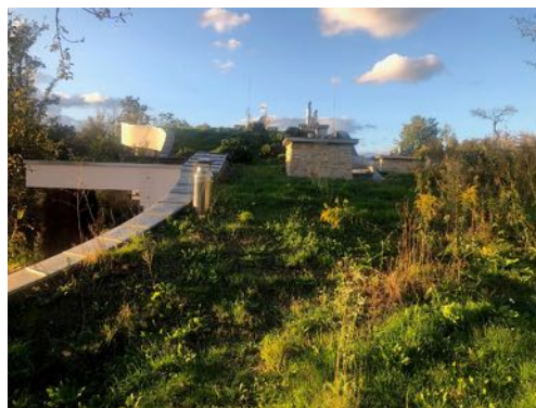
Fig. 10.: Green roof (Photo by I. Henedel)
