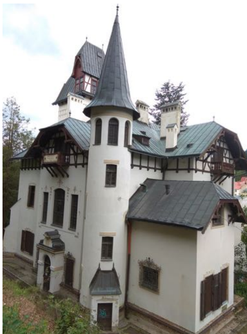
Fig. 7.: Villa Lil in Mariánské Lázně from the beginning of the 20th century, a historical building. During its life it was used as a residential villa, spa hotel, administrative building, restaurant, casino, since the beginning of the 21st century it has been empty without use. Attempts at reconstruction or sale come up against the strict requirements of the state preservation authority to preserve the authenticity of the original solution. On the one hand, this enormously increases the price of the reconstruction itself by tens of millions of CZK, and on the other hand, it makes it impossible to modify the building for such a use that would at least finance the costs of its operation. Although the building is secured, it is attacked by moisture and wood rot and gradually deteriorates. The costs necessary for its preservation and further use increase significantly every year. (Source: authors)
