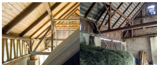
Fig. 7.: Comparison of the barn in Loubí before and after renovation (left). The planking has been replaced with carved wood. The purpose was to lighten the space, but the solution remotely resembles the ornaments of folk architecture. (Source: atelier SAD)
