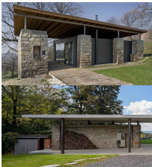
Fig. 4.: Kojetín - overall view on the first phase (top) and the second phase of the extension protecting another part of the ruins (bottom). (Source: Kamil Mrva Architects, photo: Studio TOAST)
