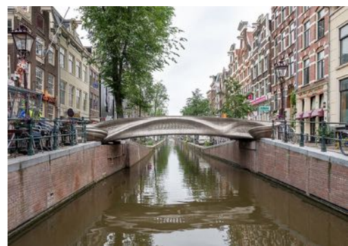
Fig. 6.: Metal bridge created using 3D printing. (Source: MX3D, 2019 Smart bridge (Source: Smart bridge, 2019. In: MX3D [online]. Amsterdam: MX3D. Available from: https://mx3d.com/industries/design/smart-bridge/ ) [Accessed June 30, 2023])
