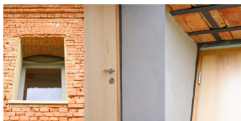
Fig. 9.: Detail of window and door openings in Arnořtov. Air gap between old and new wall is covered with a protection net. (Source: Pavel Fuchs)
