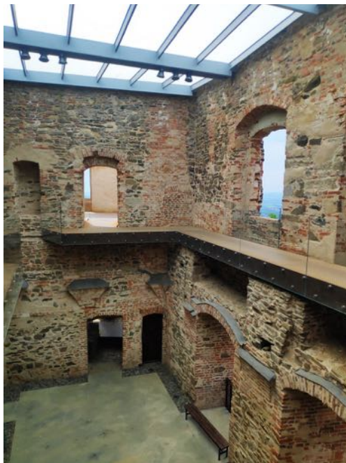
Fig. 5.: The listed ruins of Helfštýn Castle have undergone modern construction interventions that have sparked controversy and extensive debate. The static securing, safe access to the building and its partial roofing with structures made of weathering steel, concrete and glass is extremely unique and at the same time respects the torsional character of the building. In addition to the visual effect, the process of destruction of historical structures was stopped and their further life extended by several generations. (Source: authors)
