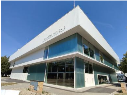
Fig. 4.: The utilitarian building of Pavilion Z at the České Budějovice Exhibition Center underwent a renovation that removed the limitations and single-purpose use of it, and achieved maximum flexibility guaranteeing its high commercial potential and thus the economic sustainability of further operation. While respecting its original material solution and layout of the exhibition area, the building was visually lightened inside and out. (Source: authors)
