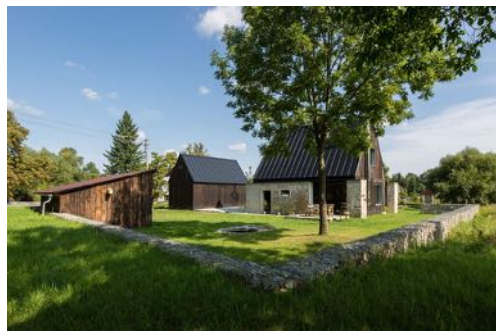
Fig. 12.: The construction of the house is inserted into the furthest part of the original building. (Source: TŘI.ČTRNÁCT architects)
