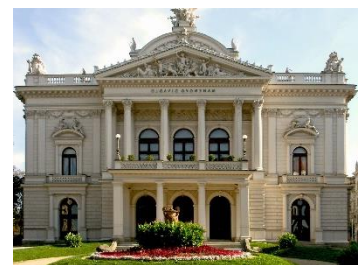
National Theatre in Brno(Fig.25)
