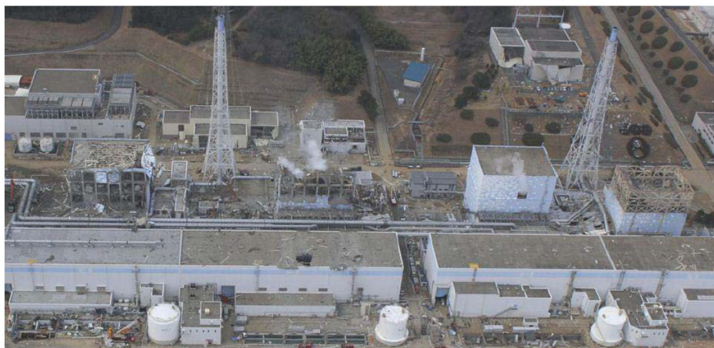
Fig.2: The Fukushima Dai-ichi NPP accident after the great Japan earthquake and tsunami in 2011
