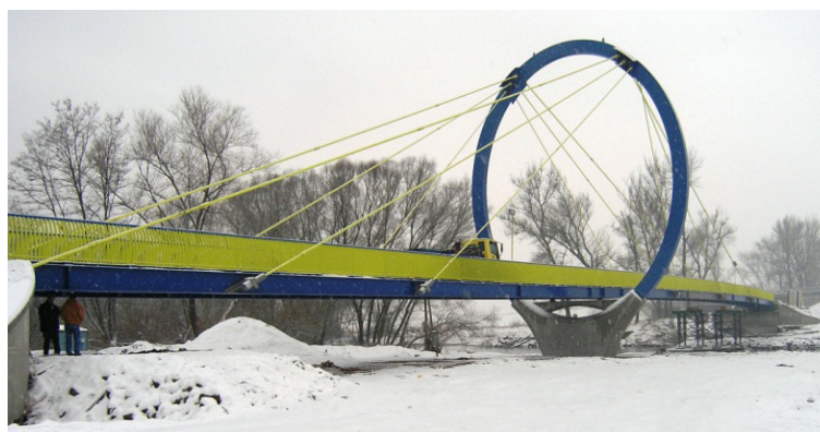
Fig. 1: General view of the cable – stayed pedestrian bridge Tennis Racket over the Hron River
