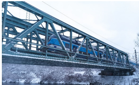
Fig. 1: Riveted steel railway bridge over the Ostravice River.
