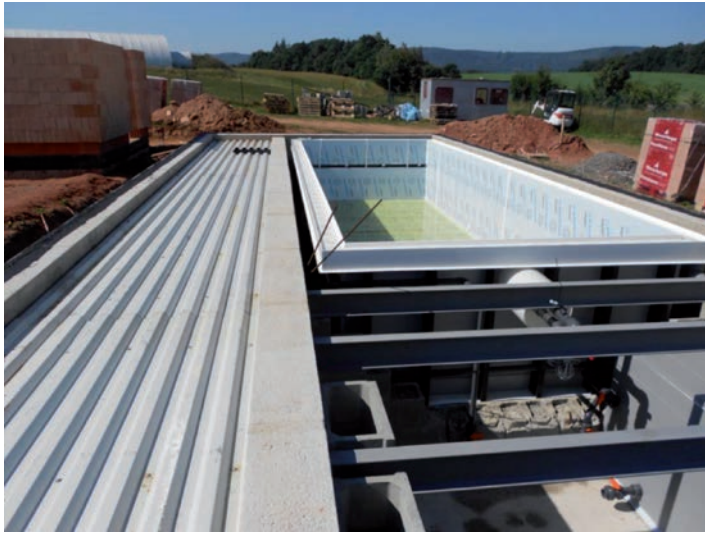
Figure. 7 Construction in August 2016. Photo: M. Nedvěď
