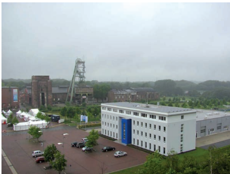
Figure.3 New construction on site Ewald in the Herten - on the roof of the new object photovoltaic panels are placed, Vojvodikova, 2011
