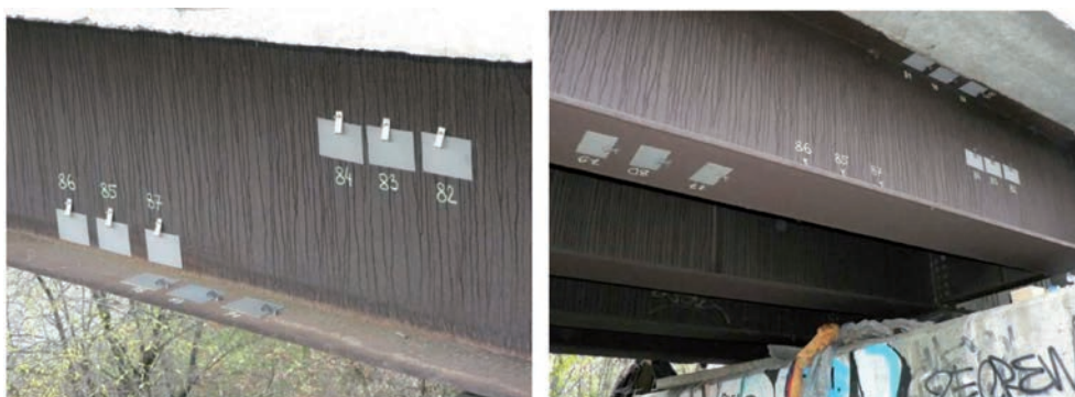
Figure 3: Installation of corrosion specimens on the railway bridge in Prague - Motol
