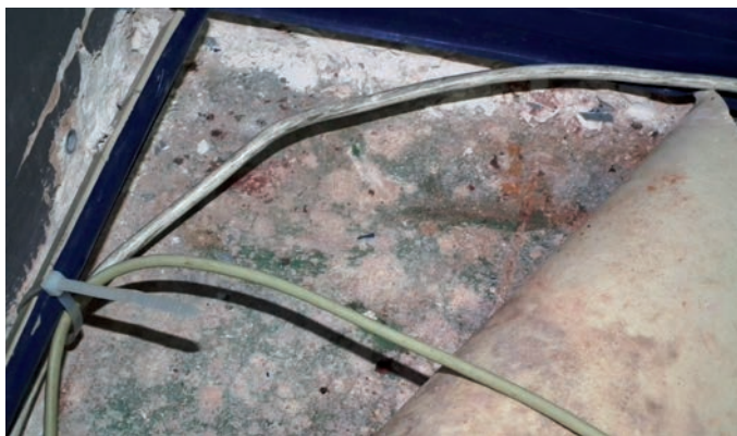
II. 1. Mould fungi occur under the carpeted floor; the ceiling over a damp cellar the most often (the author).
