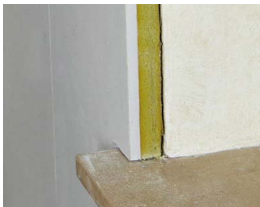
II.2. Aerial as insulation from the inside (Materials by Deutsche Rockwool Mineralwool. www.Aerowolle.de )
