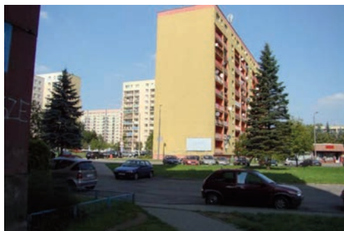
II.14. Peak wall of the building.
