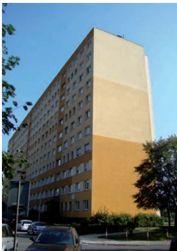
II.11. Peak wall of the building. II.
