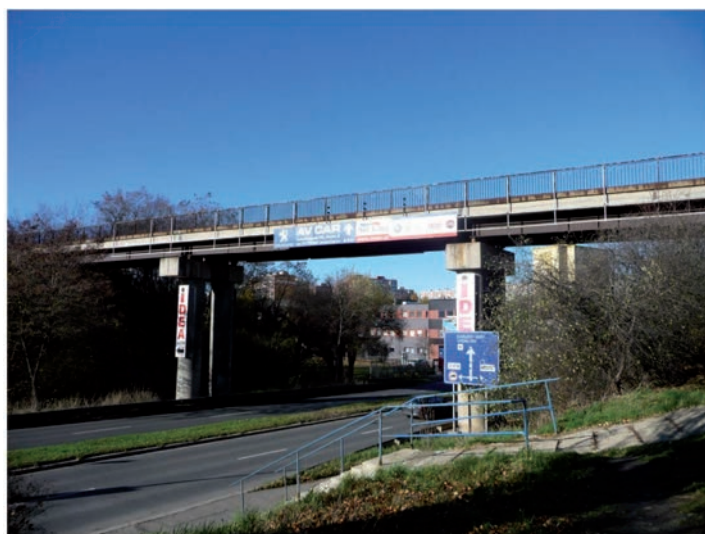
Figure 5: Side view of the railway bridge in Prague
