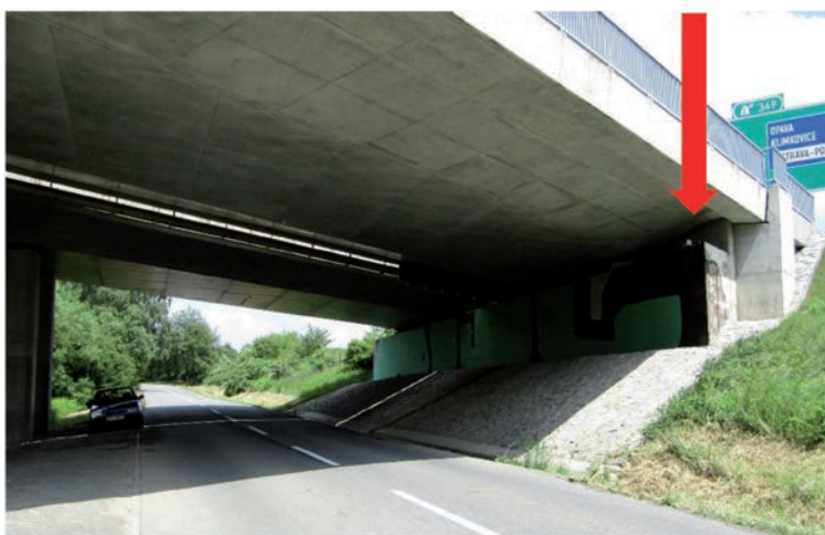
Figure 9: Concrete bridge construction across the street Vřesinská (the bridge is located below the D1)
