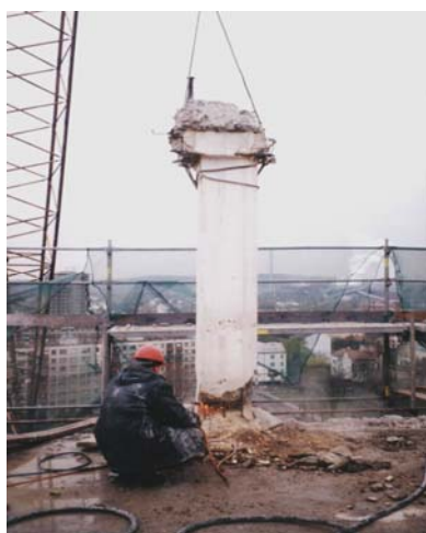
Fig. 9: Isolated columns were suspended and separated in the footing with a pneumatic hammer. the reinforcement was separated with a flame.
