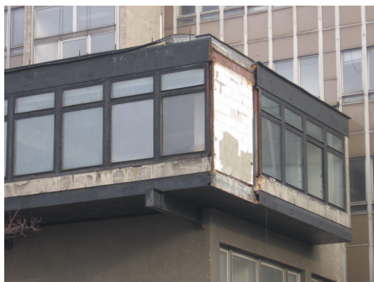
Fig. 2: Details of the facade on the administrative and office buildings ("Boletice" panels, steel skeleton, and metal windows)
