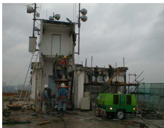
Fig. 8: A condition was (after demolition of the 14th and 15th floors) to keep the elevator shaft as well as aerials of mobile phone operators and automated control systems operated by Severomoravská plynárenská a.s.
