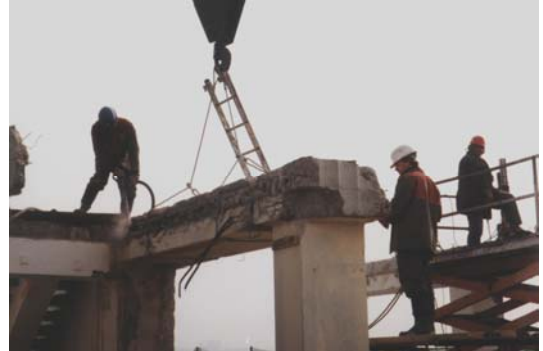
Fig. 6: All load carrying components (such as ceiling panels and girders) were drilled off in support faces. It was not possible to use another demolition method.
