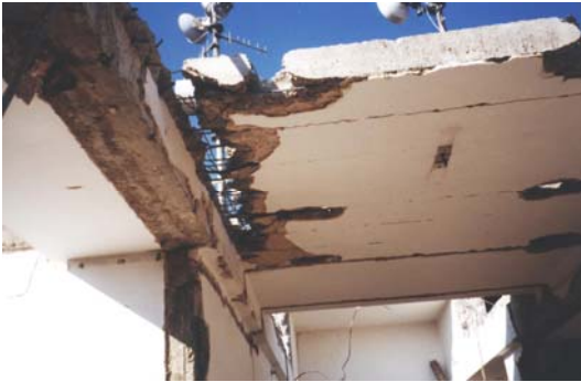
Fig. 5: PZD board ceilings in the additional storey on the roof were released from support faces
