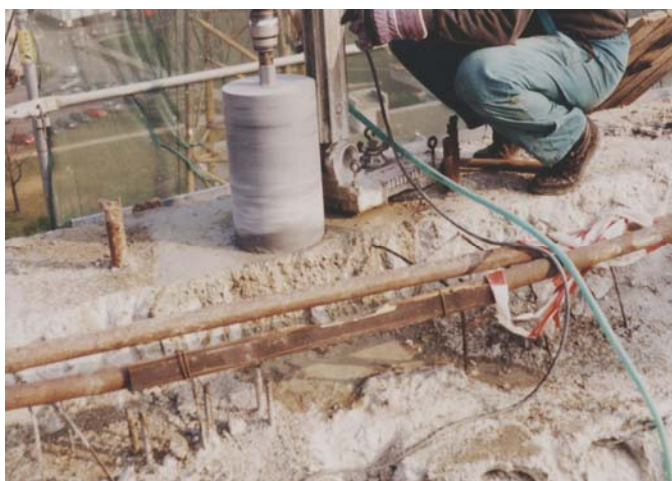
Fig. 10: The girder was drilled out to the core in the column face under the girder.
