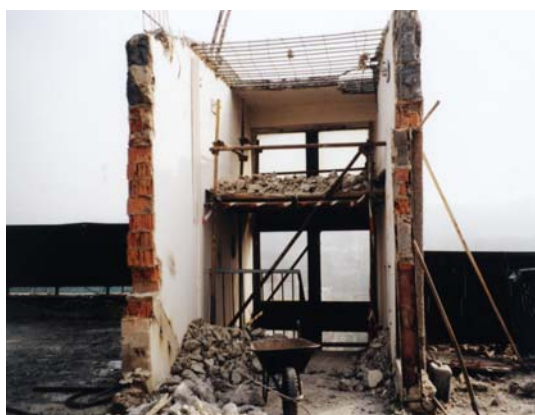
Fig. 7: After demolition of the 14th and 15th floors, the structure of the staircase remained.
