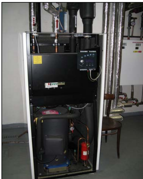
Obr. 4: TČ IVT GREENLINE F35 [4]
