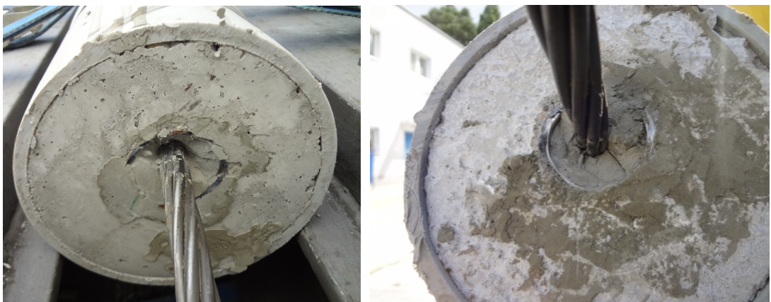
Fig. 5: Failure mode of specimens with crushed grout wedge
